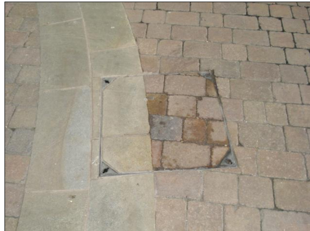
Acceptable high quality public realm utility reinstatement
