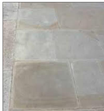
An example of high quality York Stone Paving.
