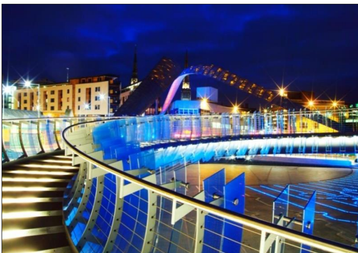
Example of a high quality and effective lighting scheme
