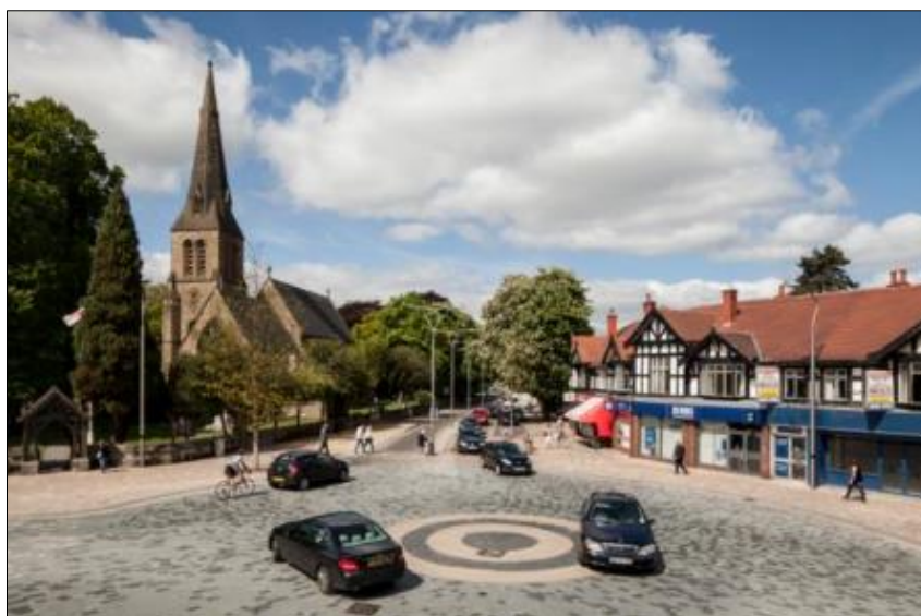
An example of a high quality shared space/street, Poynton.
