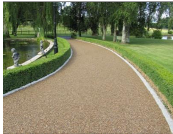
The use of bonded gravel to 'soften' tarmacadam.
