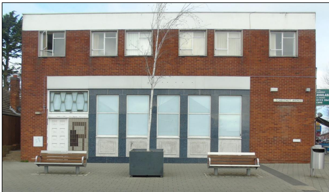
High quality, uncluttered Public Realm in Oadby core.
